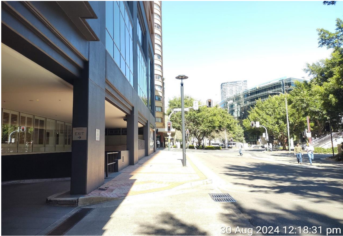
Photograph 1 Building facade, facing south
